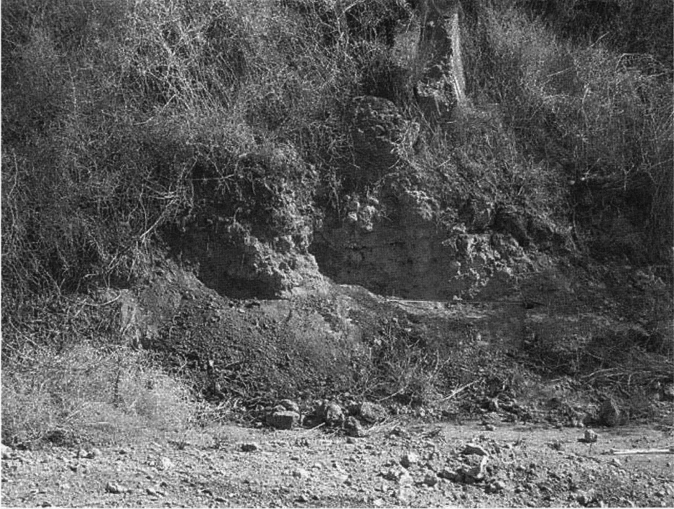
Fig. 4. Al-Maghar: a segment of the brick fortification wall, looking east
