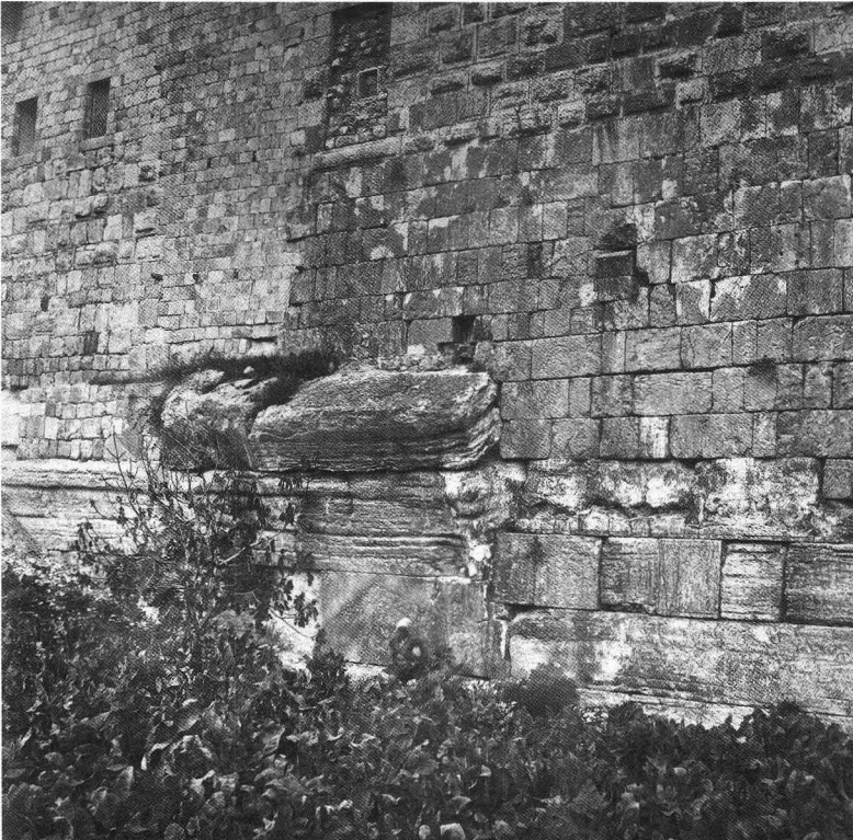
Fig. 5. The skewback of Robinson's Arch in the Western Wall of the Haram al-Sharif. Photograph taken by Sgt. James McDonald for the Ordnance Survey of Jerusalem (1864-65) (Wilson 1966, Photograph 14a = PEF/P/4297, courtesy of the Palestine Exploration Fund).
