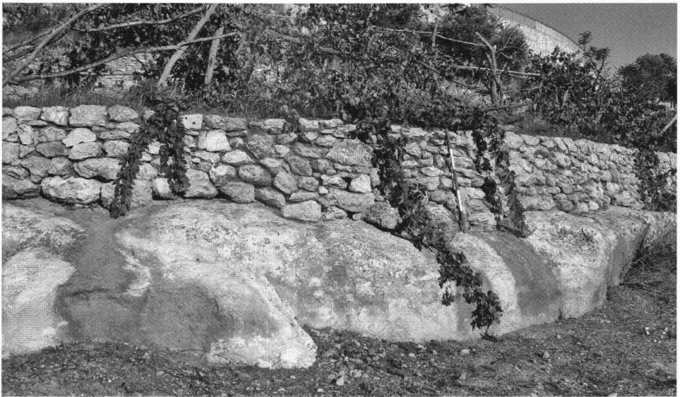
Fig. 35. Dry farm terrace drainage system at work; note water stains on rock surface
