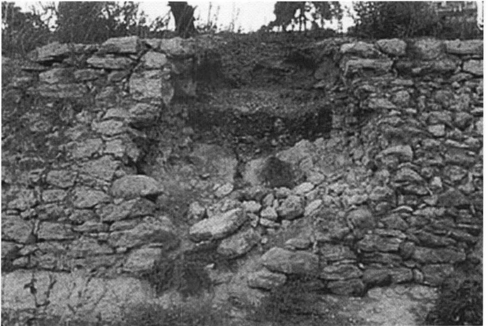
Fig. 36. Wet farm terrace F-7 constructed with layered soil
