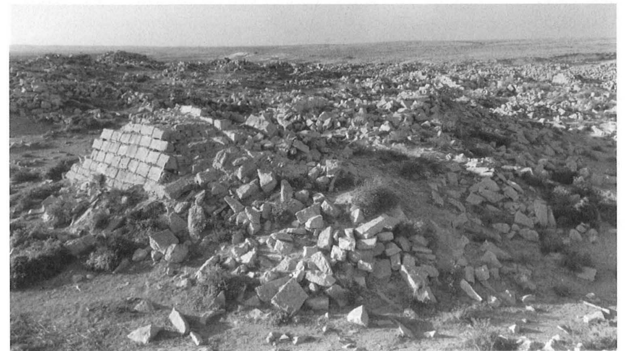
Fig. 25. Tower of House no. 2, view to the north-west
