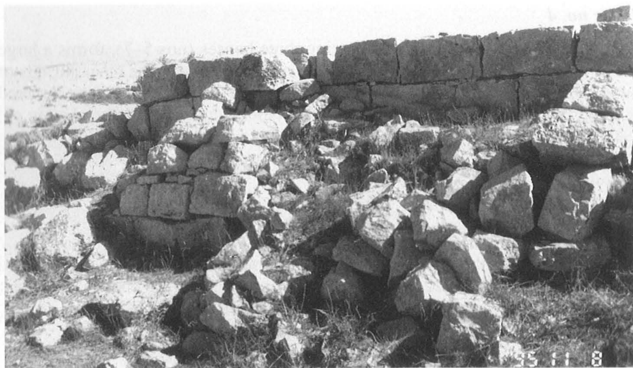
Fig. 26. Sloping retaining wall along House no. 8, view to the north-east
