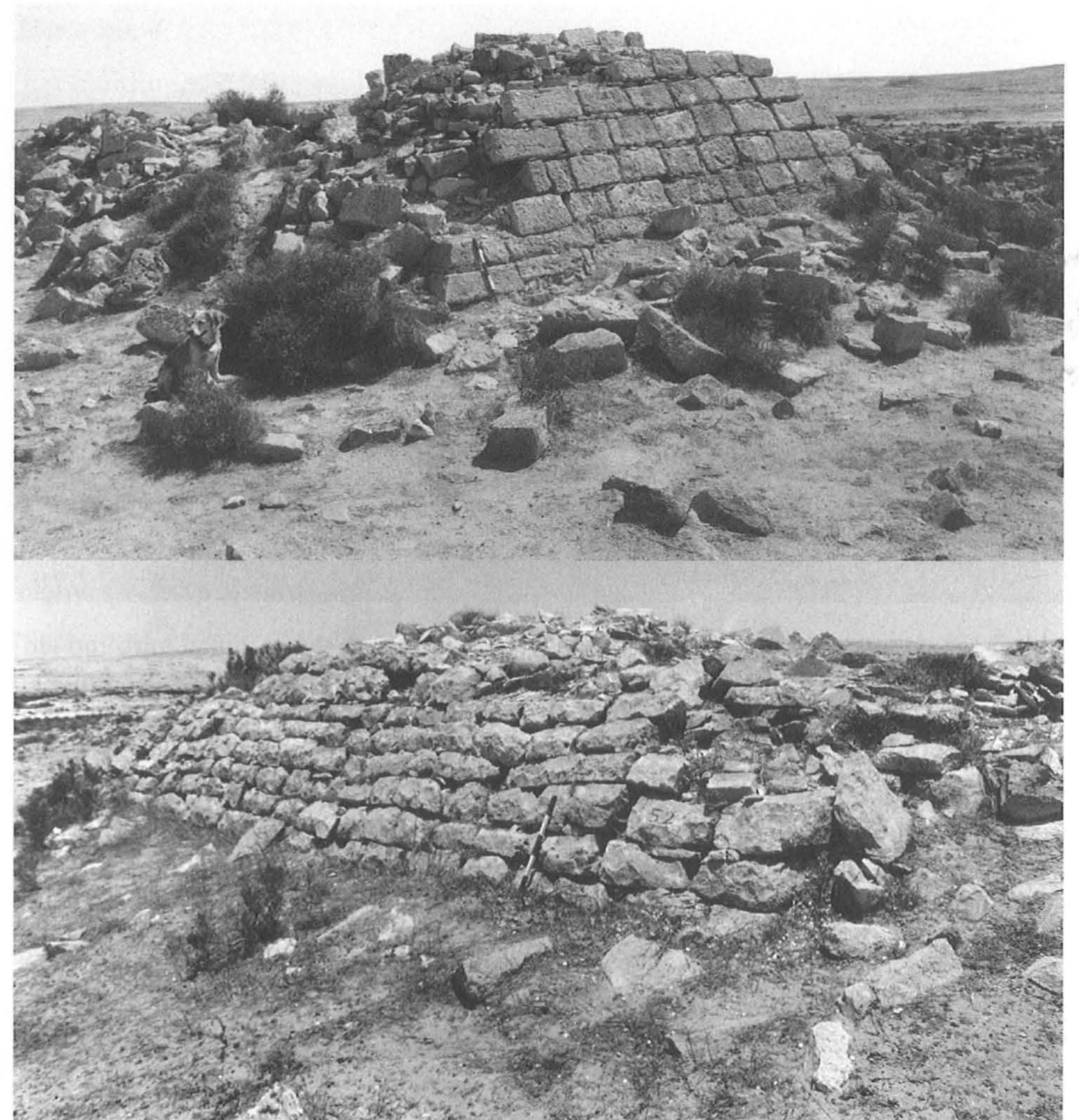
Figs 22 and 23. Two types of retaining walls characterizing construction at Sa'adon
