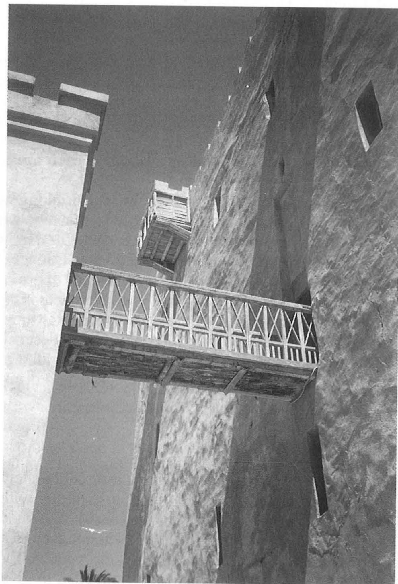
Fig. 10. Deir Abu Makar: Drawbridge enabling access from belfry on left to tower (Photo C. Dauphin).
